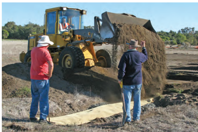
Roy dumps the 'fill' on top of the shade cloth covered metal
