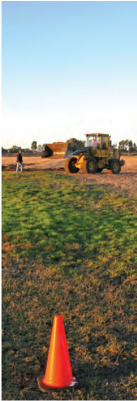
More pics from the Drain Fill Project
